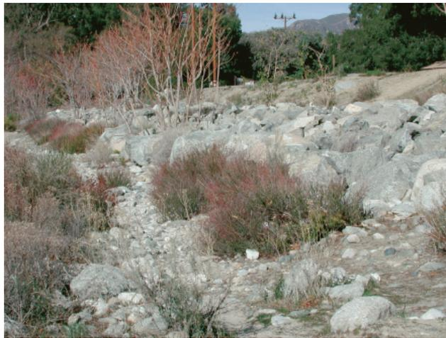
Figure 18—This area was filled to build a parking lot (flat area in upper right) and the bank was stabilized using riprap.
