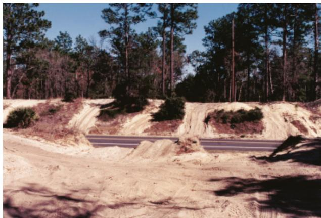
Figure 36—Damage caused by OHV use on the Ocala National Forest.
