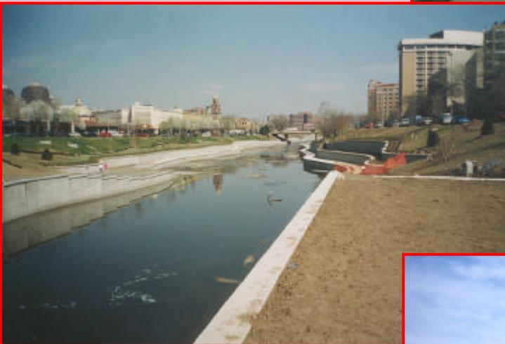
**C**onstructed stream channels are often designed for flows greater than bankfull. Normally, this type of channel is too wide to efficiently move sediment during flows at bankfull or less. These channels usually require high construction and maintenance cost.
