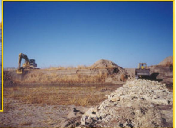
**B**endway weirs and rock vanes are constructed as a group extending along the length of an eroding area. Individual weir length, width, upstream angle and spacing between weirs varies from site to site and structure to structure.
