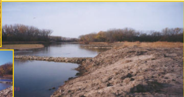
**R**educed water velocities on the downstream side of bendway weirs result in sediment deposition near the bank.
