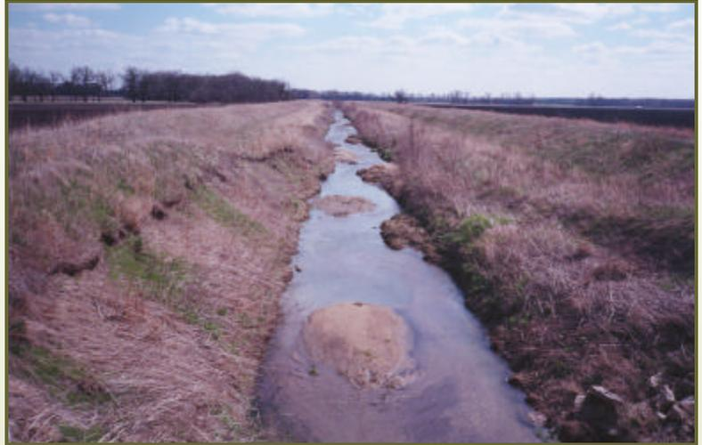
**A**s headcuts move upstream, the deepening channel remains narrow with high water velocities. Eroded material is transported downstream where water velocity slows due to a wider or meandering channel with a flatter slope. When water velocities are reduced, excess sediment is deposited, constricting the channel and increasing flood problems.
