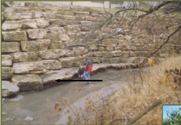
**T**he arrows in these pictures indicate stream bed elevations at the time each structure was constructed. The stream channels have since lowered, or incised, due to changes in the stream or watershed.
