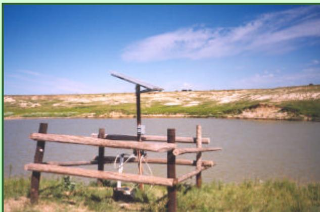
**T**he systems pictured at right and below, utilize submersible pumps in wells. This type of system is suitable for use throughout the year.
