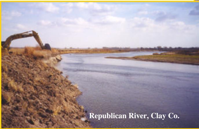
**V**ertical streambanks must be shaped to provide a suitable surface for planting cuttings, seedlings, and grass. On large stream systems, structures such as **ROCK BENDWAY WEIRS** or **ROCK VANES** should be installed prior to vegetative planting. (see page 36)
