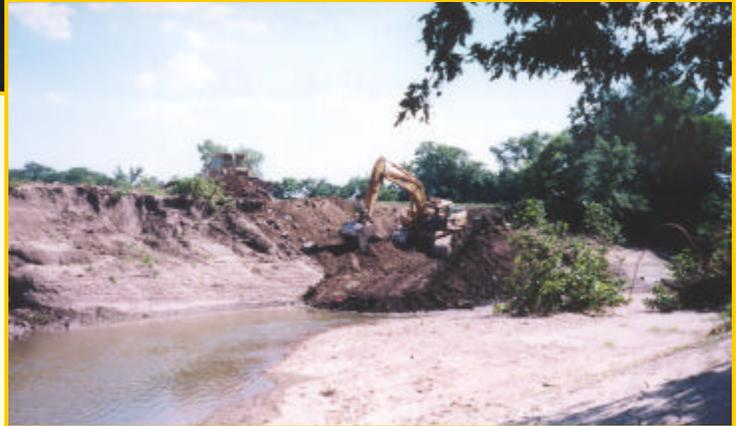
**T**he same site immediately after bank shaping and installation of 4 rock vanes.
